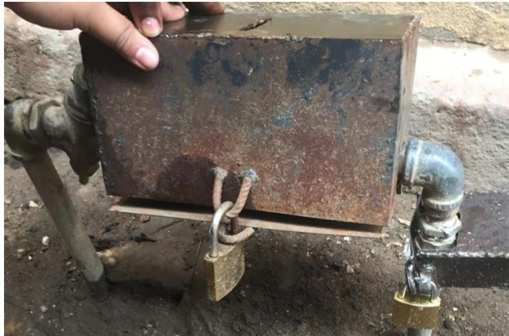
**Figure 1.** Steel case and pad-lock to control water availability to tap-users. *Source:* Author's original
