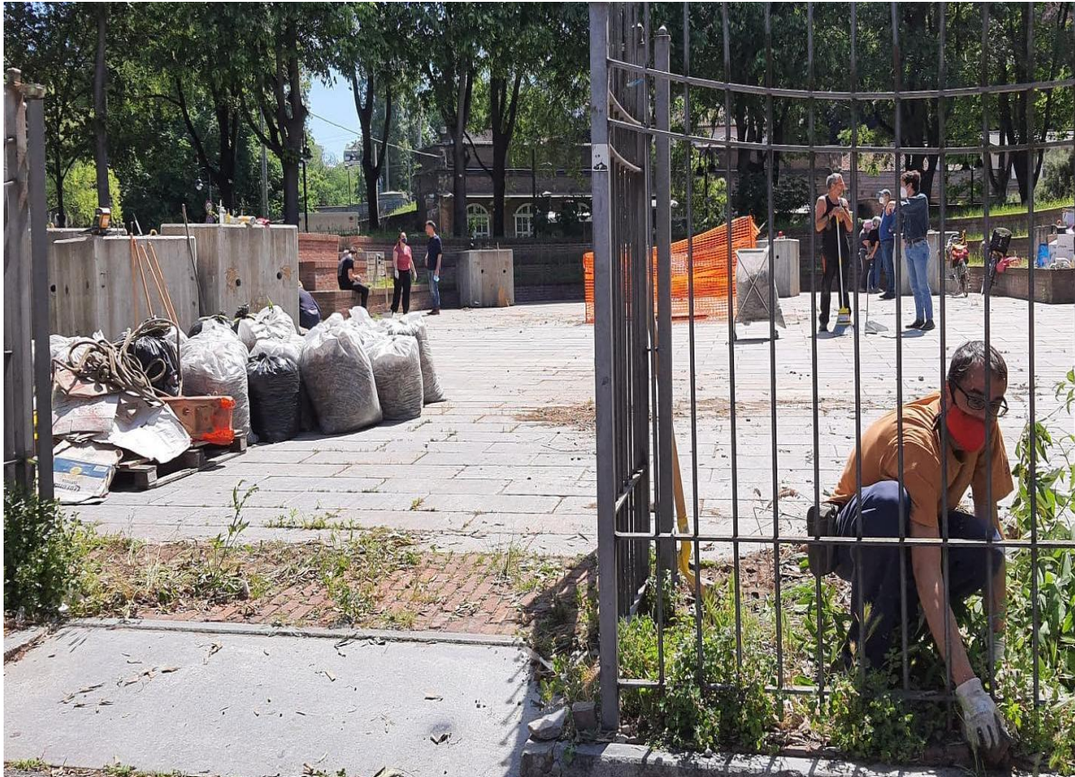
Figure 3. Collective work to re-open the Giardino Pellegrino (credits: FCPP)
