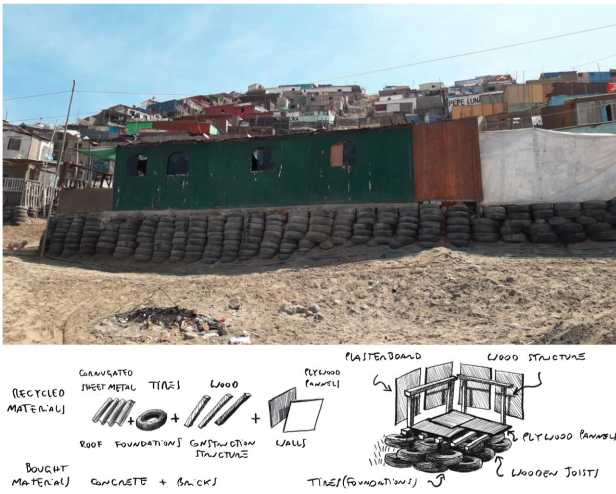
Figure 9. Urban mining and reuse of objects and materials is an observable part of the construction of houses. Photo and graphic elaboration by the author, 2018
