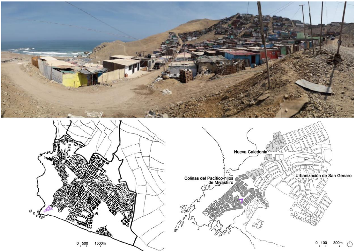
Figure 4. Above: view of the Asentamiento Humano Colina del Pacífico-hijos de Miyashiro . Below: Asentamiento Humano within the Chorrillos district and plan sketch. Source: author's elaboration, 2024
