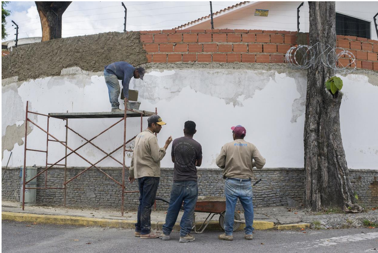
Figure 3. Construction of additional layers on existing perimeter wall. Photo by Edgar Martínez
