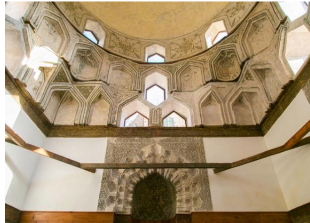
Figure 16. 'Shajar al-Durr's' mausoleum after being restored. (Source: Megawra, n.d.)
