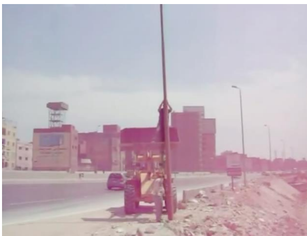
Figure 8. The community installing the lighting posts. (Source: Elnaggarism, 2012)
