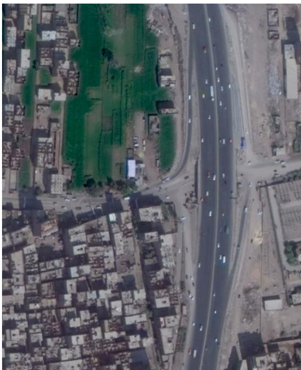
Figure 6. The ring-road after building the exits. Source: Google Earth V7.1.5.1557. (July 5, 2015). Giza, Bulaq. 30° 03' 01.93"N, 31° 10' 37.66"E, Eye alt 655 feet. DigitalGlobe 2012. http://www.earth.google.com [April 26, 2012].
