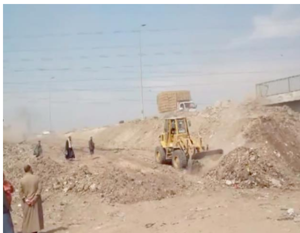
Figure 7. The work in process. (Source: Elnaggarism, 2012)
